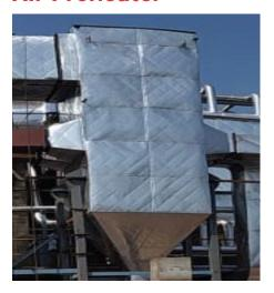
Our advanced Airpreheaters excel at heat transfer, preheating the combustion air using the heat from the flue gas. By raising the temperature of the incoming air, these accessories significantly enhance combustion efficiency, leading to improved fuel utilization and reduced energy consumption.
